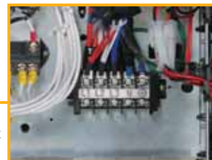
Outdoor unit power supply terminal block
