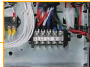
Outdoor unit power supply terminal block
